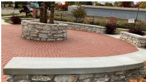
The major ground's project was the instillation of a concrete cap on the 47-foot, semi-circle limestone wall in the sculpture garden around the plaza. The cap was needed to prevent further deterioration of the limestone during the winter. All limestone is from the original depot foundation. The cap also provides more comfortable exterior seating.
